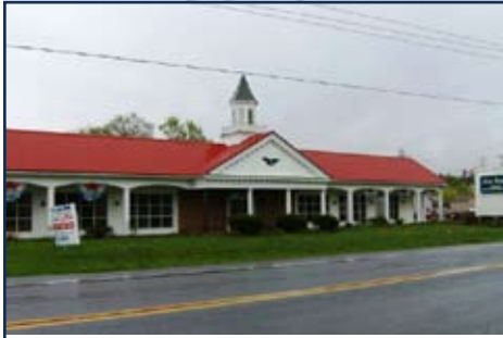
375 N Greenbush Office/ Retail Space 14,400 SF can subdivide
