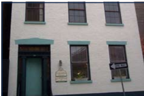
48 Columbia Street, Albany Office Space Up to 1,650 SF
