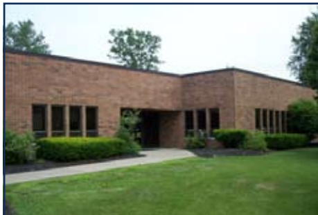
26 Computer Drive South, Albany 11,787 SF $775,000
